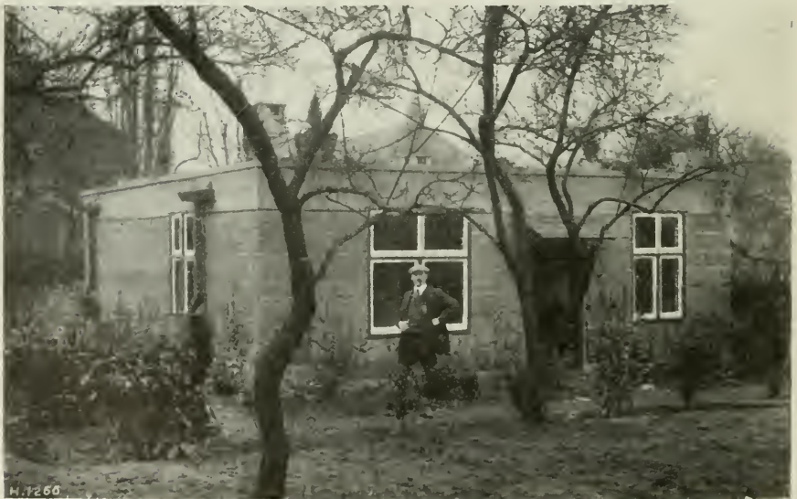
FIGS. 37 AND 38.—CONCRETE COTTAGES ERECTED ON MESSRS. ROWNTREE'S ESTATE.
